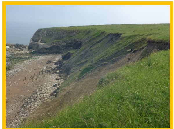
Slippage in cliff at Chemical Beach (/0106C01)
