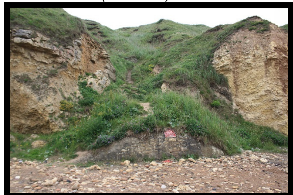
Closed access steps (/0301C01)
