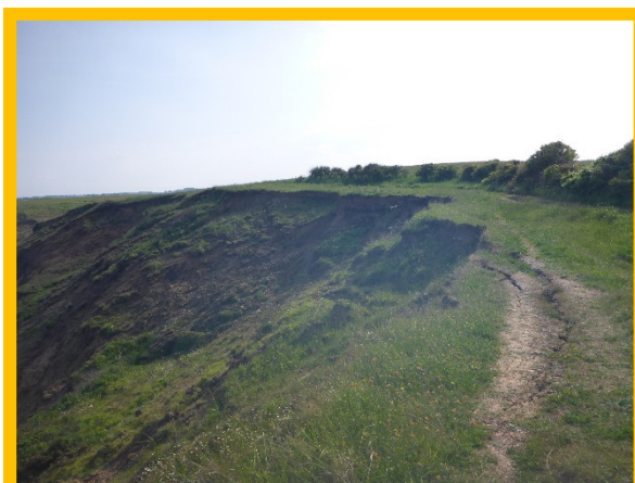
Tension cracks in path at cliff top (/0201C01)
