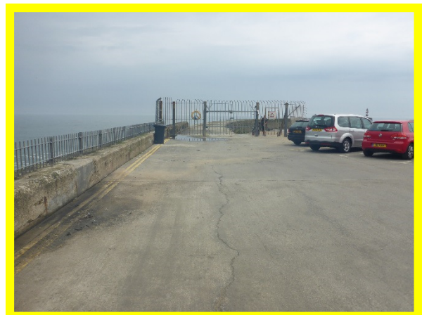
Deck of Seaham Harbour North Pier (/0104C03)
