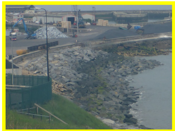
Tipped rubble (/0104C16) and rock revetment (/0104C01)
