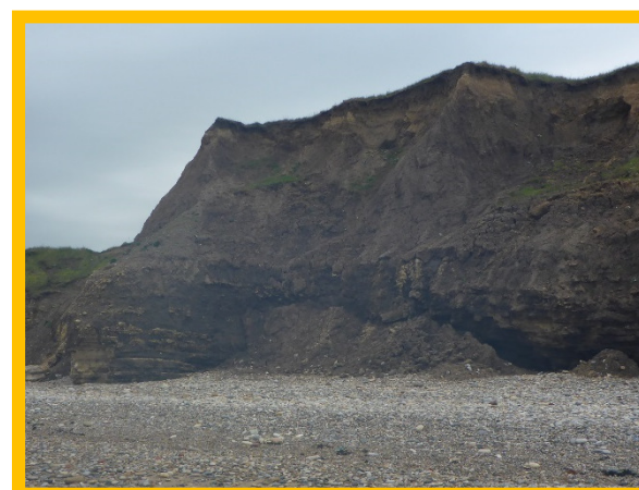
Localised slumping of upper till within the cliffs (/0804C01)
