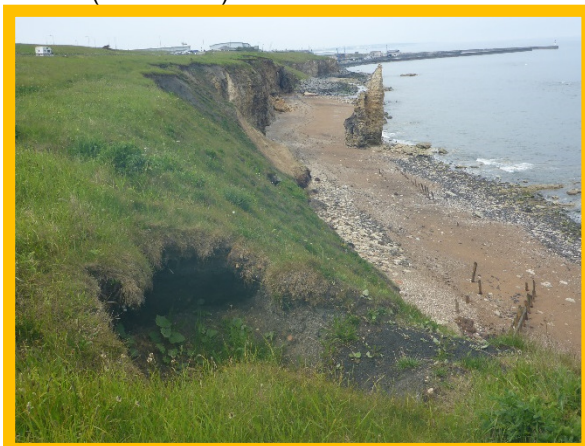
Recent slumping at headscarp (0106C01)
