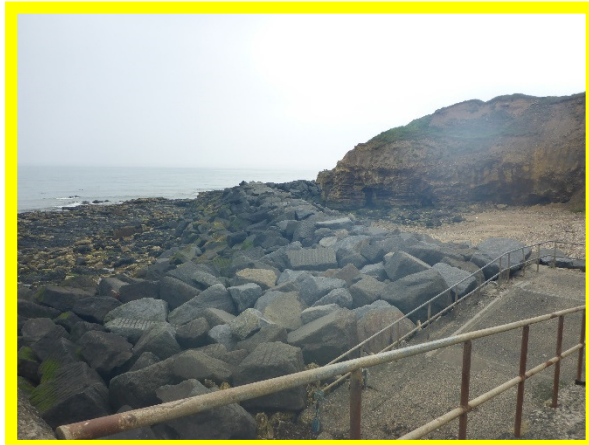
Rock berm around Featherbed Rocks headland (/0103C01)
