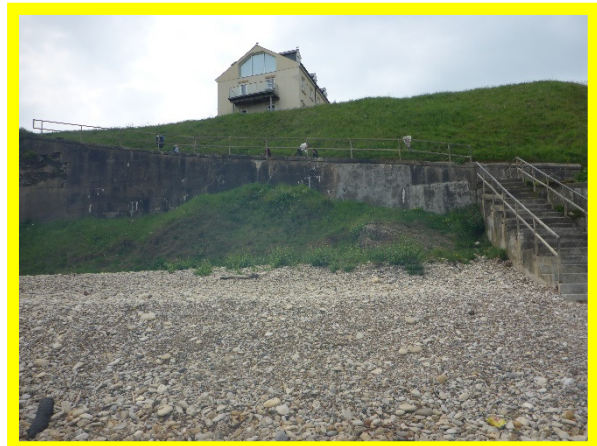
Access ramp and steps (/0103C07)
