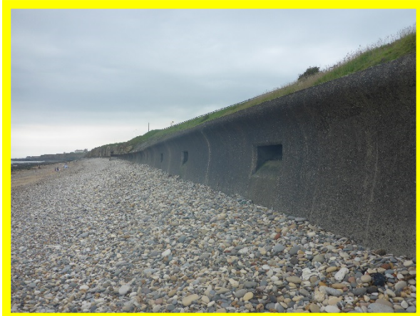
Seaham sea wall (/0102C01)
