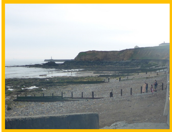
Remnants of groynes (/0102C01)
