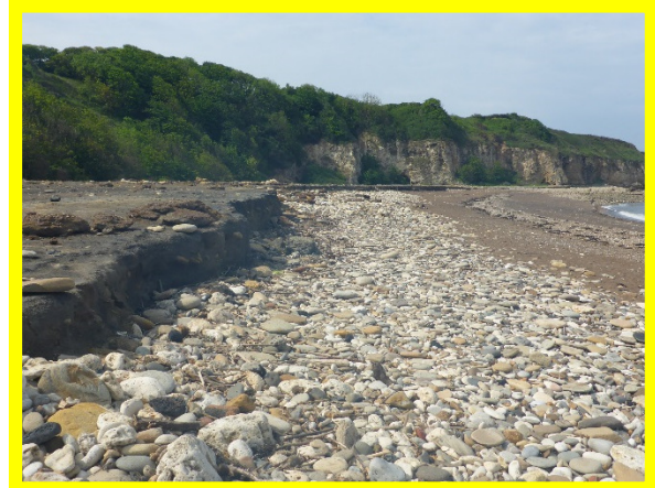
Residual spoil beach at Hawthorne Hive (/0201C01)
