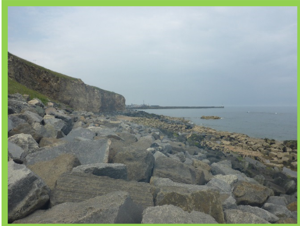
Rock revetment from South Pier to Chemical Beach (/0105C01)
