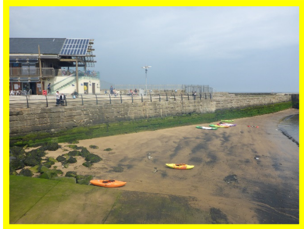
Several damaged/chipped blocks (/0104C06)
