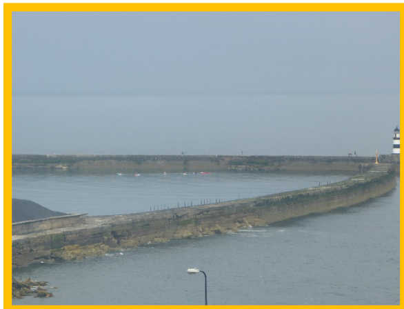
Seaham Harbour South Pier (/0104C17)
