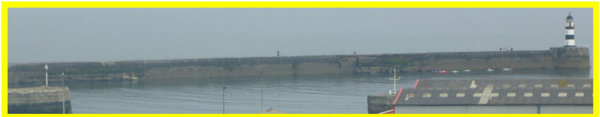
Seaham Harbour North Pier Inner Face (/0104C03)
