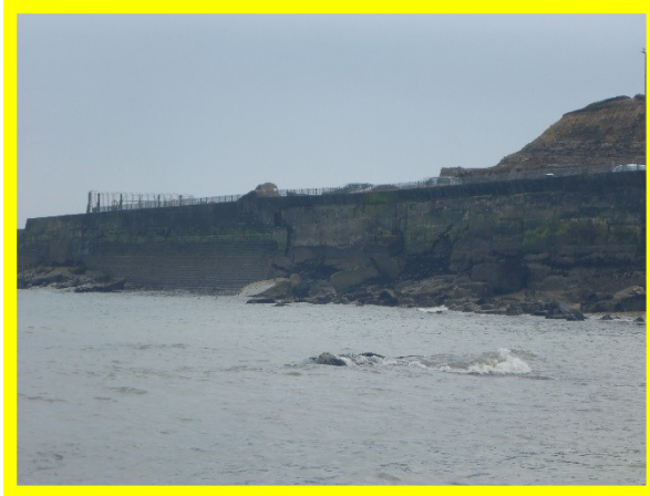
Seaham Harbour North Pier Outer Face (/0104C03)
